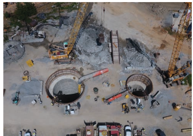
Right: Aerial view of primary and lower level pump station shafts
